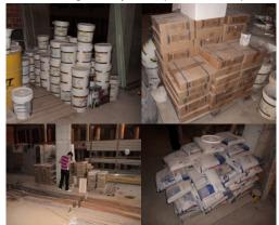
Figure 2. Above and left: stack of buckets texture, top right: stack of boxes pellets; below and to the left: stack of boxes of tiles and PVC pipes to the bottom, bottom right: stack of bags of mortar.
